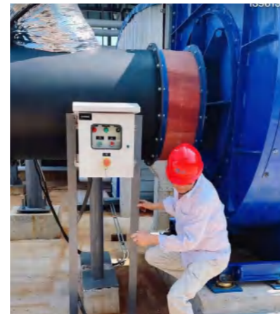
On-site Inspection Conducted at GCL ET
