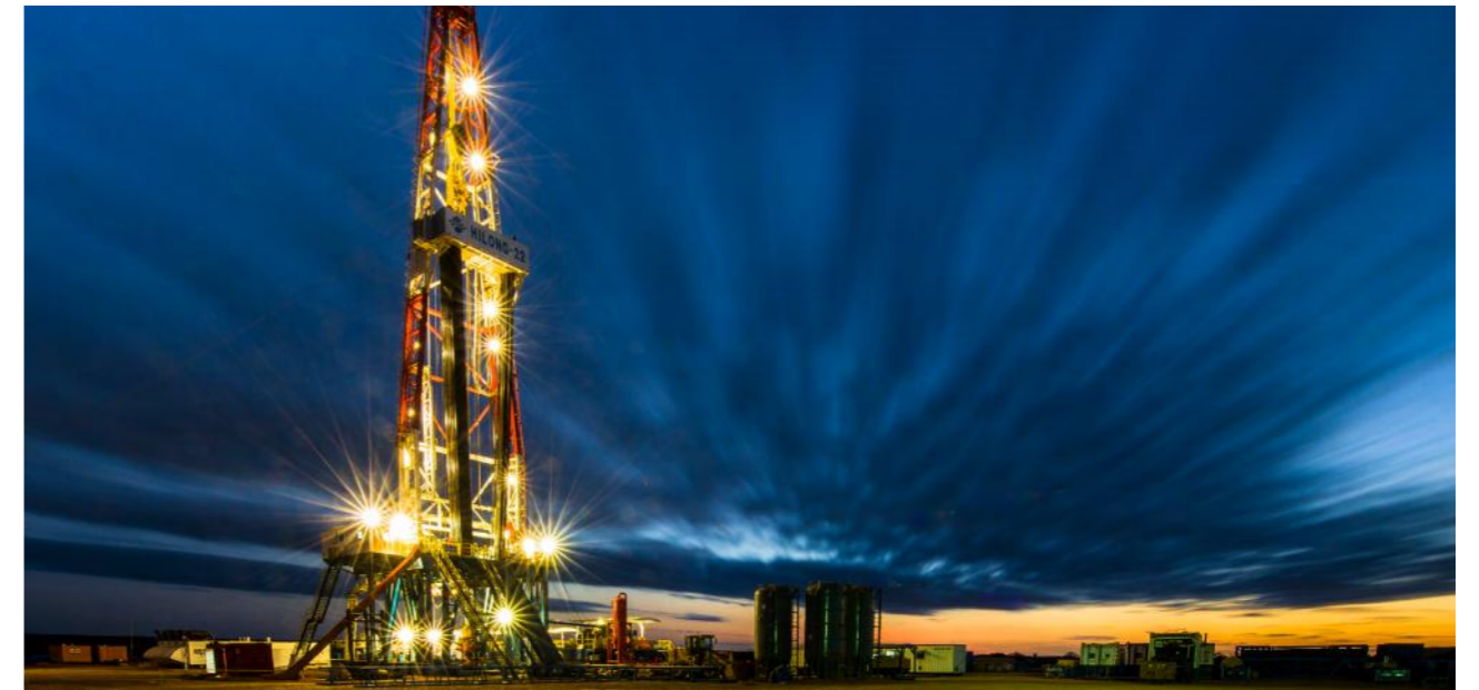
A Natural Gas Project in Ethiopia
