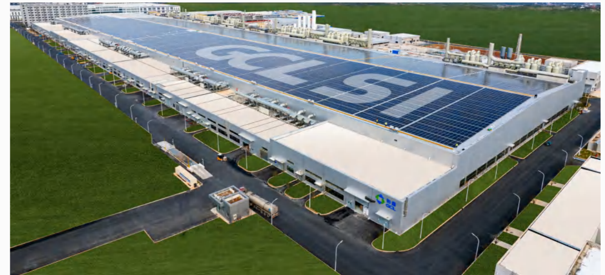
Wuhu GCL Photovoltaic Power Station
