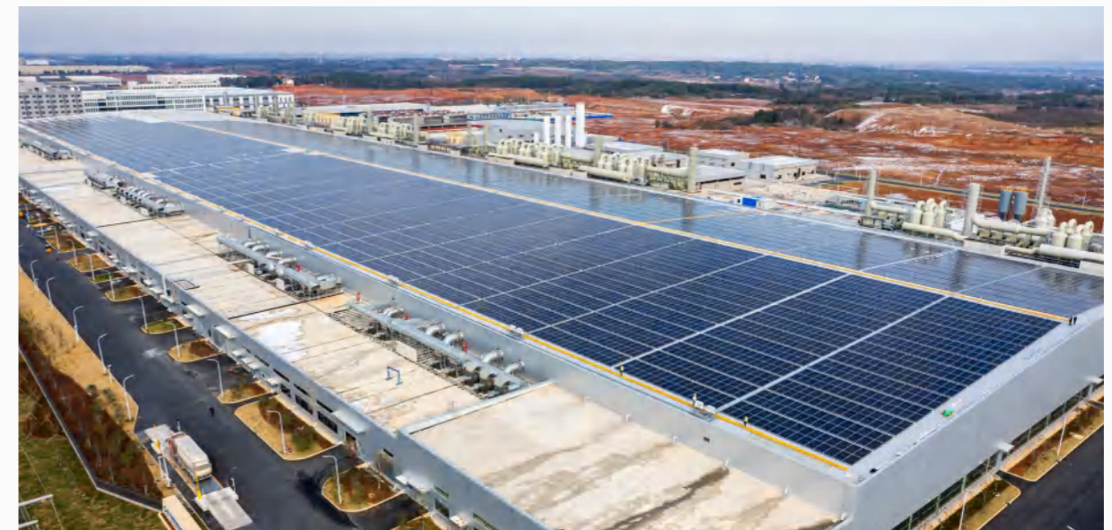
GCL ET Distributed Photovoltaic Power Generation Project
